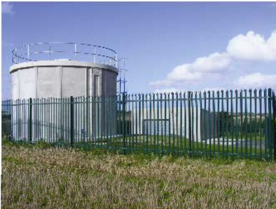
Photograph 1-1: Sheepgrange Group Water Scheme in County Louth, which was upgraded in 2012 with a new reservoir and treatment facility.
